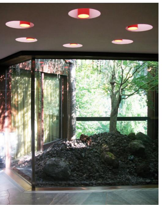
light: small circular light wells allow plenty of natural daylight in most of the rooms. to experience this feeling of being showered in light in the evening or on darker days, artificial light is integrated in these wells. long metal tubes are positioned on the inner surfaces of these cylinders. these new elements are coloured bright red or green creating an optical illusion. architecture becomes op-art.
